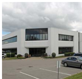
1401 Courtneypark Dr E 53,496 SF Toronto West
